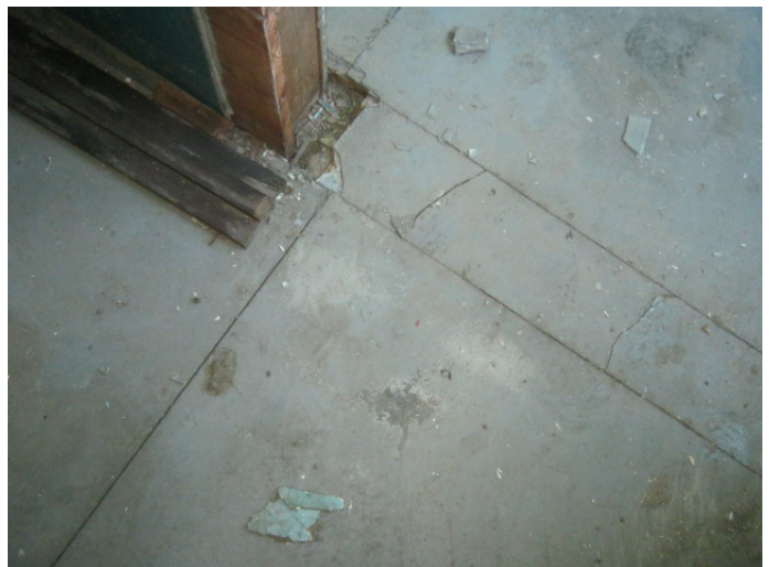
Asbestos-cement board flooring observed in 2 nd floor bath. (Sample set 22)
