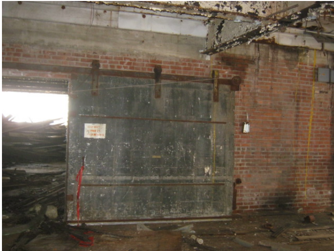
One of several PACM fire doors observed throughout the Main Mill Complex.
