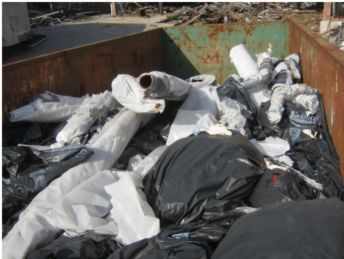
Previously abated ACM inside roll-off dumpster onsite. Dumpster reportedly removed prior to this report.
