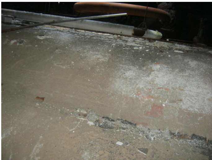
Asbestos-containing jacketing on oil-fired boilers. (Sample set 32)
