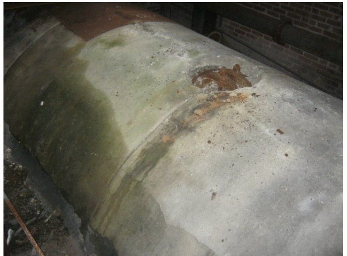
Asbestos-containing jacketing on wood-fired boiler. (Sample set 31/PACM)
