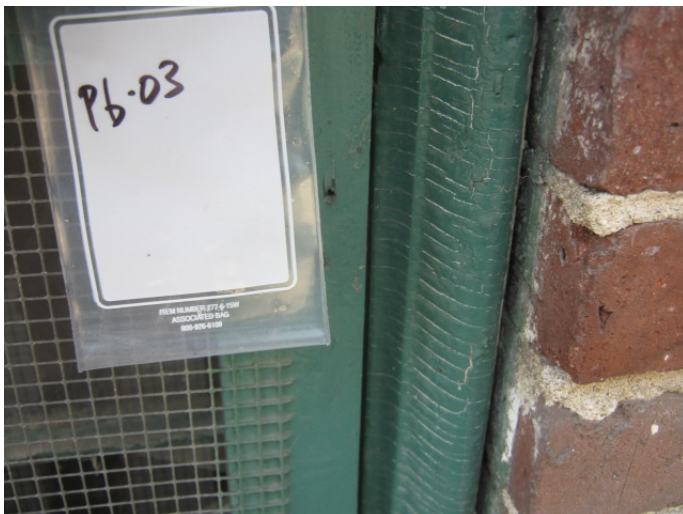
Lead-based paint on exterior window components on Main Mill Building exterior.
