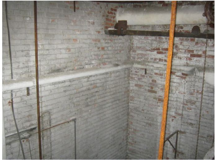
Large- and small-diameter asbestos-containing pipe insulation observed inside boiler room. (Sample sets 28, 33)
