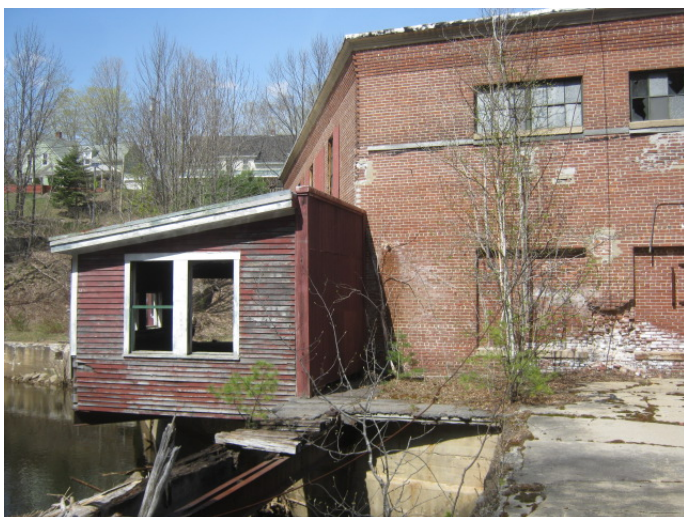
View of "rear wood addition" including windows with ACM glazing. (Sample set 06)
