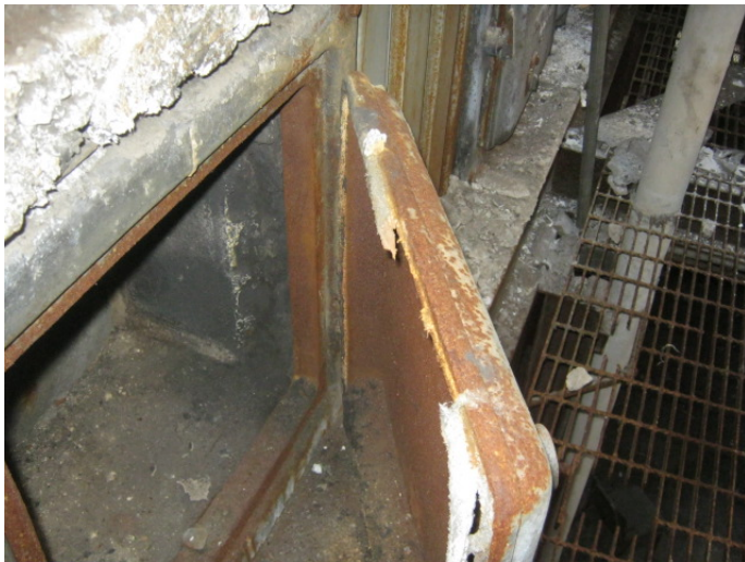
Asbestos-containing gasket observed on one of three boilers. (Sample set 30)
