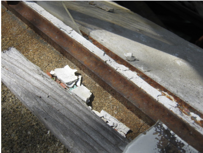
Closer view of ACM window glazing on “partial demo section” steel sash windows.
