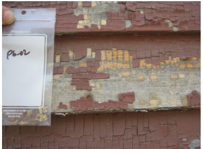
Lead-based paint on wood clapboards on Main Mill Building exterior.
