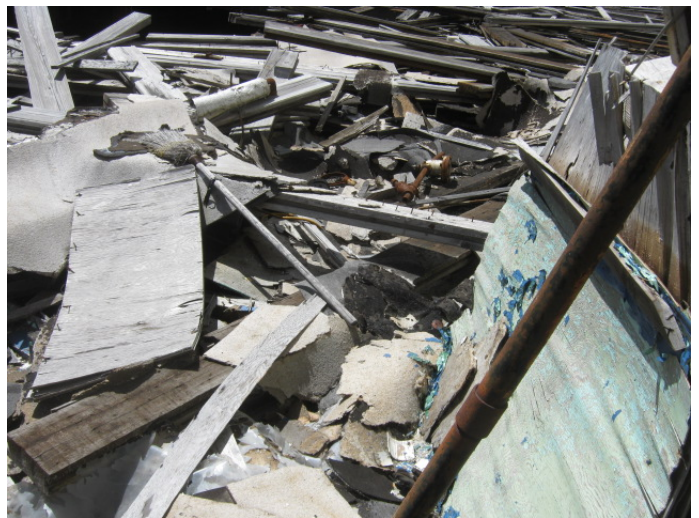
PACM asphalt-containing roofing mixed in with demolition debris at Site.
