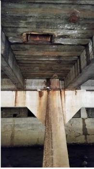
Photo 26: View of an approximately 2' x 1' hole in the floor of the main mill building which leads directly to the river. Note cast iron outfall/discharge, and stormwater outfalls in background.
