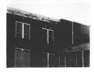
Photograph 22 – Deterioration of Eave and Roof, Northwesterly Area of Building Complex
