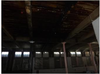
Photo 101: Black oily staining of the ceiling of the first floor of the Site building.
