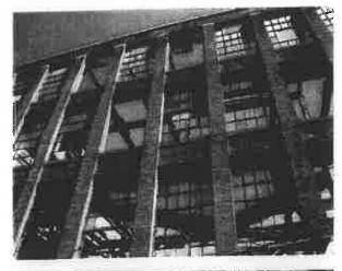
Photograph 38 – Deterioration of Brick in Southerly Masonry Wall
