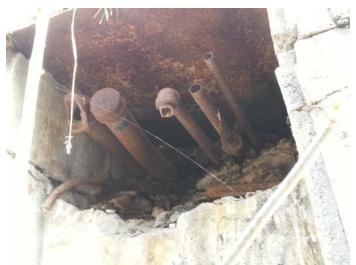
Photo 43: Piping associated with the former 100,000-gallon oil storage bunker in the northwestern portion of the Site.
