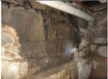
Photo 75: Area of significant oil staining on walls in the central portion of the Site building basement (former manufacturing area).
