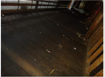
Photo 121: Black staining on the floor of the storage area in the eastern portion of the third floor of the Site building.
