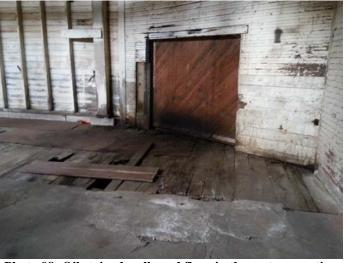
Photo 98: Oil stained walls and floor in the eastern portion of the first floor of the Site building.
