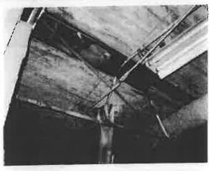
Photograph 57 – Holes in Floor Due to Water Intrusion below Area Shown in Photograph 55
