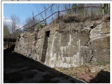
Photo 41: Former 100,000-gallon oil storage bunker in the northwestern portion of the Site. View is to the northwest.
