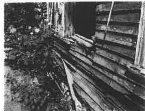
Photograph 32 Floor Framing Resting On Exposed and Deteriorated Column above Area Shown in Photograph 30
