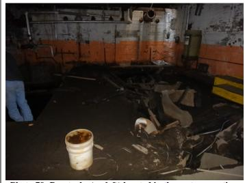
Photo 79: Penstocks (on left) located in the eastern portion of the Site building basement. Standing water remains.
