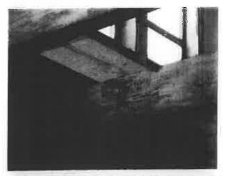
Photograph 53 – Deterioration of Floor Framing and Flooring Due to Water Intrusion
