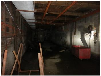
Photo 77: Hallway in the eastern portion of the Site building basement. Piping along the concrete wall to the right is capped fill and vent pipes for a former oil storage tank.
