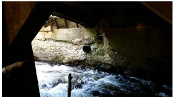
Photo 28: Outfall/drains which discharge directly to the stream from the main mill building, typical.
