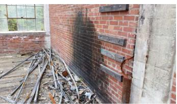
Photo 116: Oil-stained walls observed in the partially-demolished portion of the second floor of the Site building.
