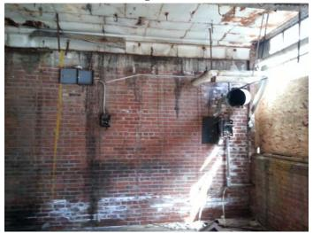
Photo 89: Oily staining observed on the floors and walls of rooms in the central/northern portion of the Site building basement.
