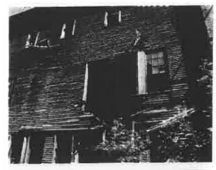
Photograph 29 – Open Hole in Roof of an Auxiliary Building
