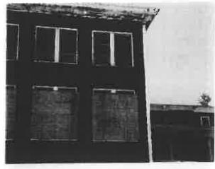
Photograph 20 – Deterioration of Eaves on Northerly Side of Building Complex
