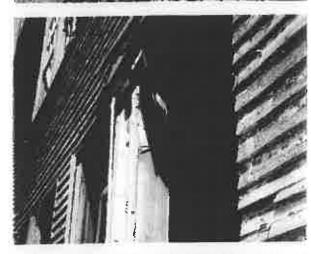
Photograph 33 – Four Story High Masonry Wall Standing on Southerly Side of Site with Floors Removed
