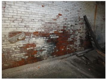
Photo 99: Oil stained walls in the eastern portion of the first floor of the Site building.
