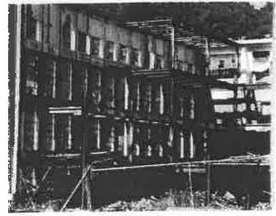
Photograph 34 – Masonry Wall Section with No Lateral Support
