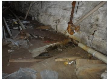
Photo 67: Another view of trench drains discharging to a common sub-surface drain.
