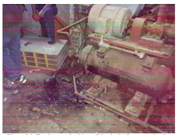
Photo 94: Equipment leaking oil in the boiler room in the eastern portion of the Site building basement.
