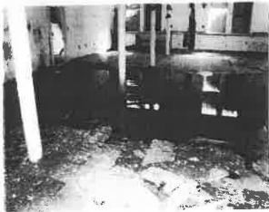
Photograph 49 – Deterioration of Floor Framing Due to Water Intrusion
