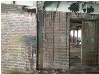
Photo 88: Oily staining observed on the floors and walls of rooms in the central/northern portion of the Site building basement.
