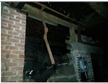
Photo 76: Second area of significant oil staining on walls in the central portion of the Site building basement (former manufacturing area).
