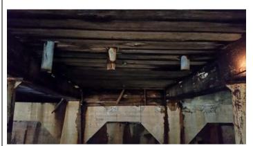
Photo 27: Outfall/drains which discharge directly to the stream from the main mill building, typical.
