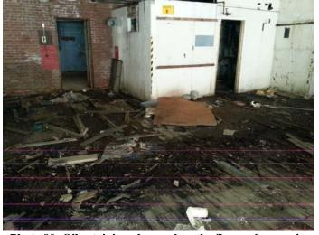
Photo 90: Oily staining observed on the floors of rooms in the central/northern portion of the Site building basement.
