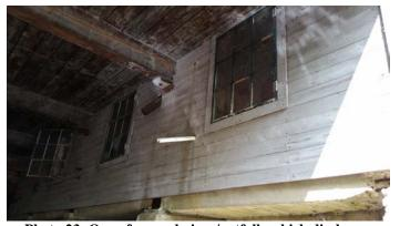
Photo 23: One of several pipes/outfalls which discharge directly to the stream from the main mill building.
