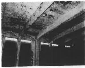
Photograph 47 – Water Leaking through Roof of Main Building Complex
