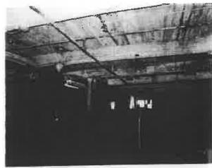
Photograph 56 – Portion of Roof Collapsed into Second Floor above Area Shown in Photograph 55
