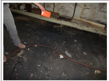
Photo 69: Oil-stained floors observed in the eastern portion of the Site building basement (former printing room).
