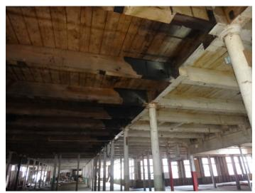
Photo 100: Black staining on ceiling of the first floor of the Site building.
