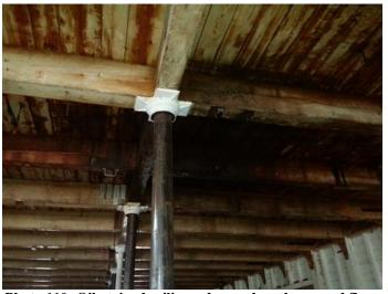
Photo 110: Oil-stained ceilings observed on the second floor of the Site building.
