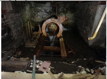
Photo 85: Turbine located in the northeastern portion of the basement of the Site Building. Evidence of dumping in the open water surrounding the turbine.
