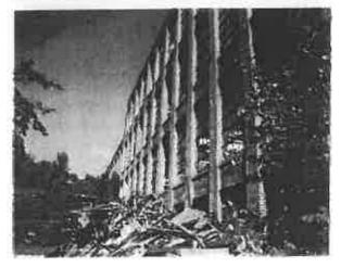
Photograph 37 – Windows Missing from Southerly Masonry Wall
