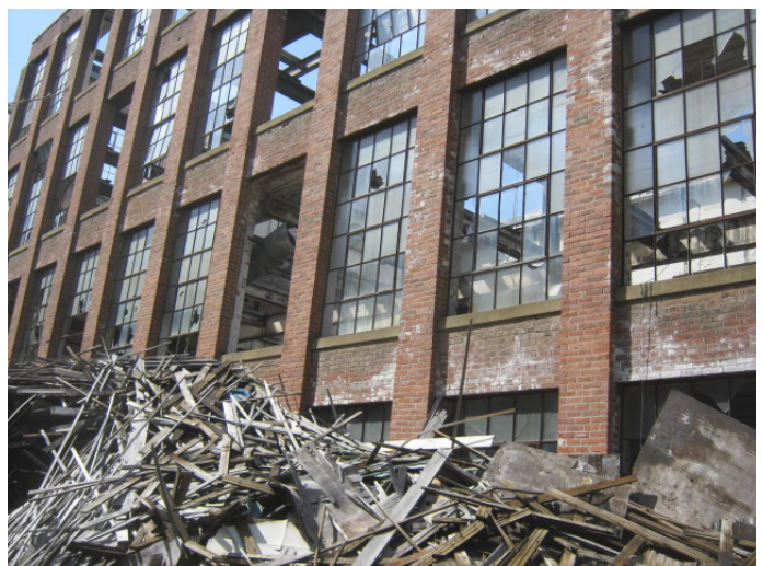
Steel sash windows with ACM interior glazing on "partial demo section." (Sample set 09)
