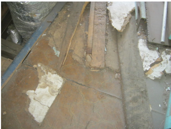
Brown sheet flooring observed in 1 st floor bath. (Sample set 16)
