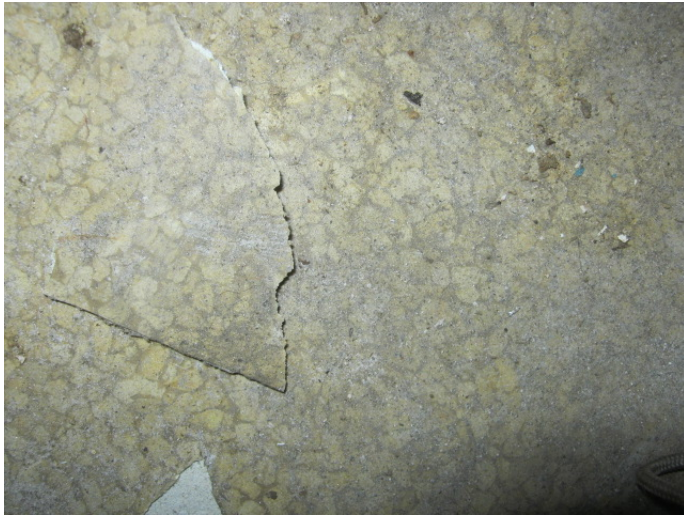
Pebble pattern sheet flooring observed on Main Mill Building 2 nd floor. (Sample set 26)
