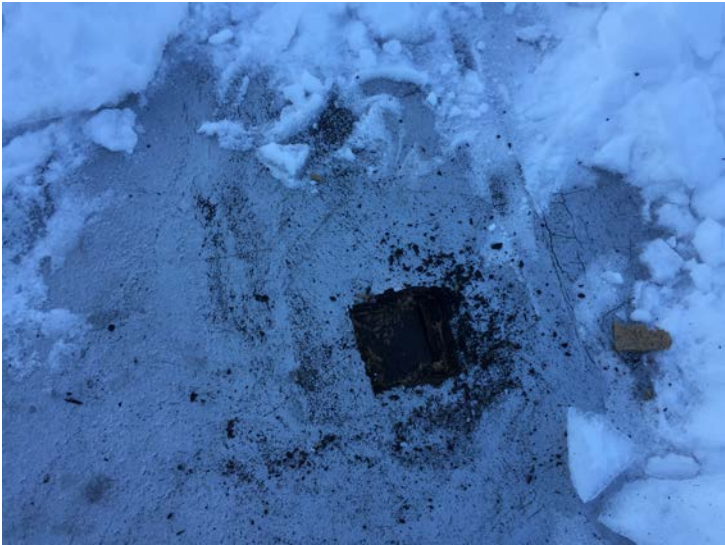
Closer view of core cut sample with silver coat, asphalt roll roofing, over tar & gravel "built-up" roofing. (Sample E2).
