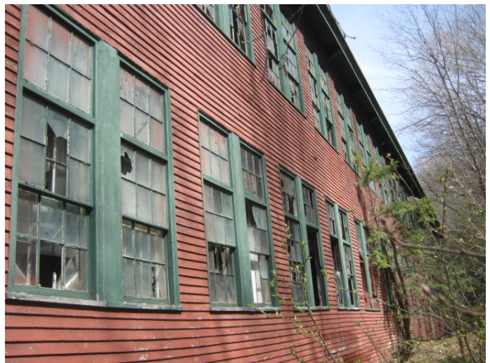
View of several windows on Main Mill with ACM glazing. (Sample set 03)
