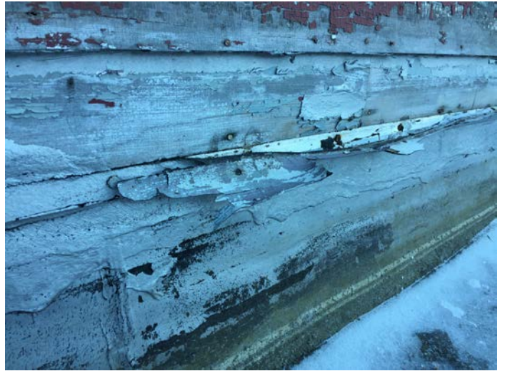
Silver coat sealant, observed applied to the large majority of roofing areas (Sample set SCS).
