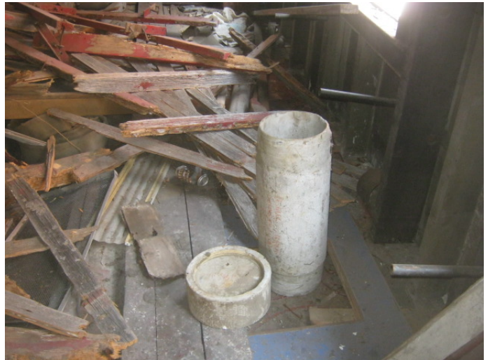
Asbestos-cement piping and cap observed inside Photo Building. (Sample set 01)
