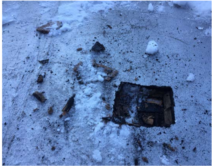
Closer view of core cut sample with only asphalt roll roofing, coated with silver ACM sealant (Sample D)
