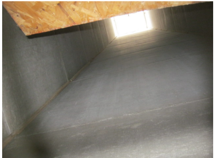
Asbestos-cement paneling lining vertical shaft on Main Mill Building west exterior wall. (Sample set 14)
