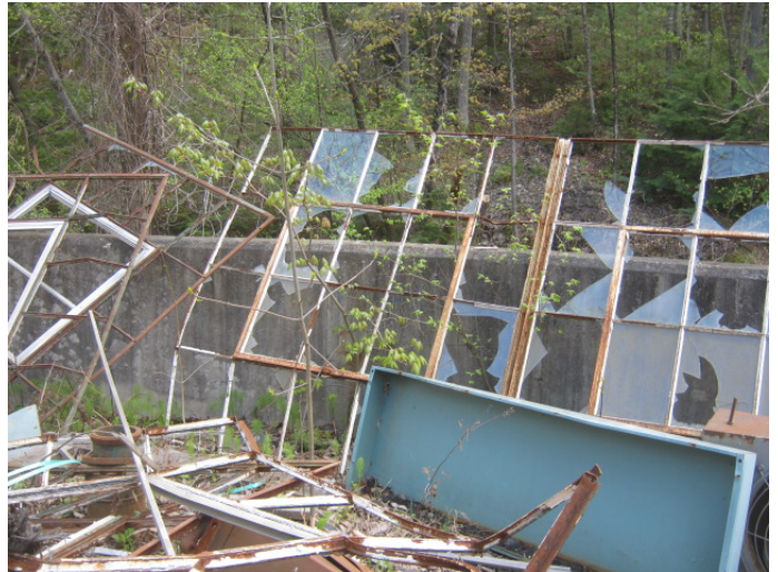
Steel window sashes presumed from "partial demo section," removed from building and mixed with demolition debris.
