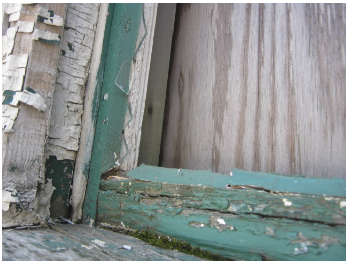
Exterior window glaze on Main Mill Building wood-sash windows. (Sample set 02)
