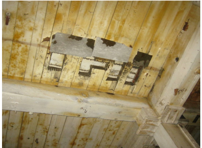
Small pieces of asbestos-cement board nailed to ceiling in Main Mill Building. (Sample set 12)
