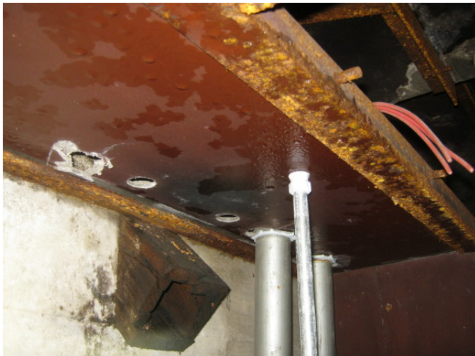
Asbestos-cement paneling inside electrical room in Main Mill Building basement. (Sample set 13)
